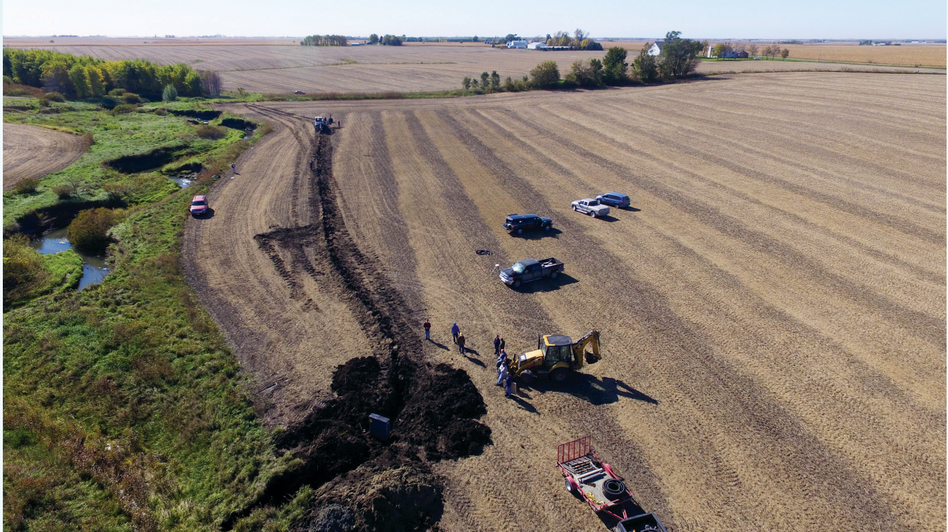
Saturated buffer installation
